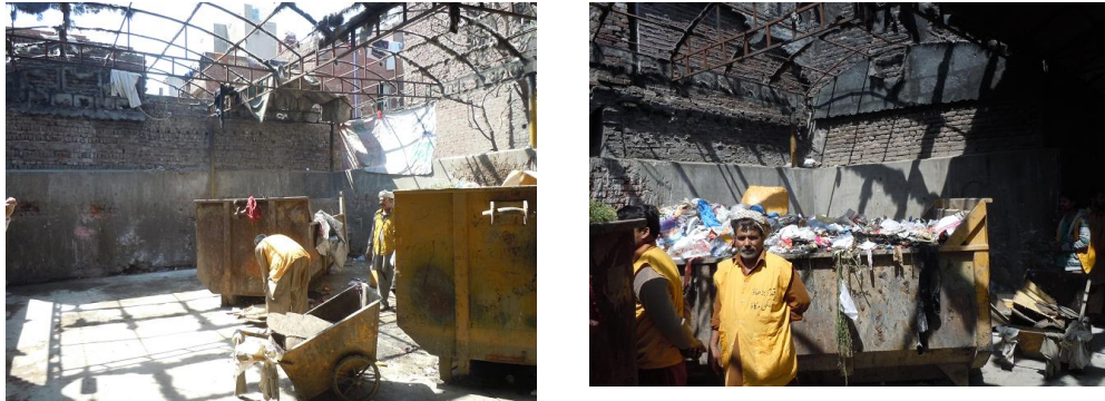
Photo 2.3.2 Current Situation of Waste Collection in Khali Transfer Station
