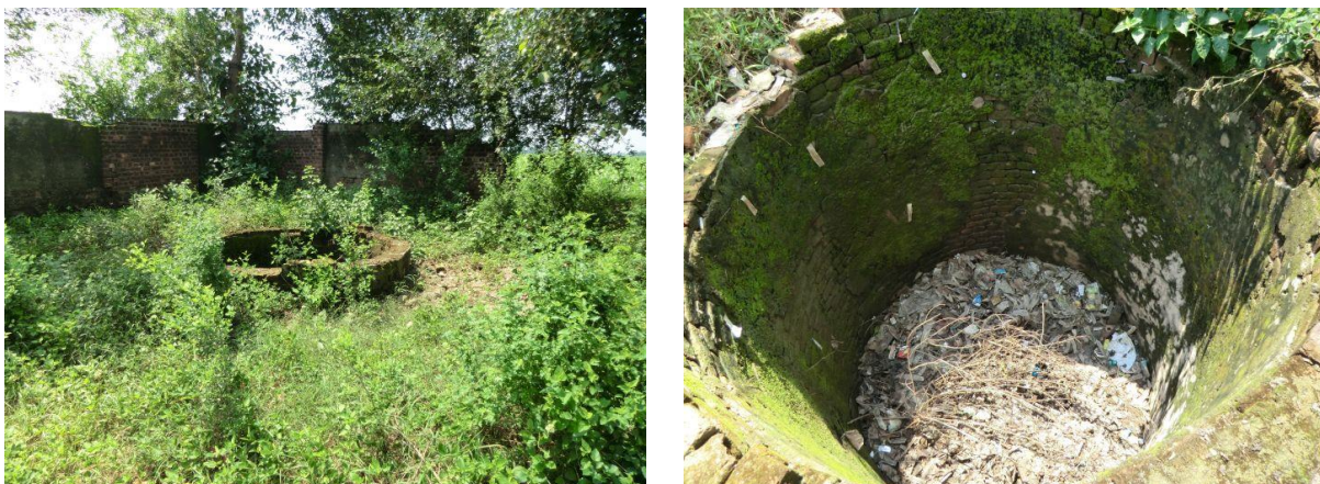
Photo 2.10.3 Pit for Risk Waste at BHU
