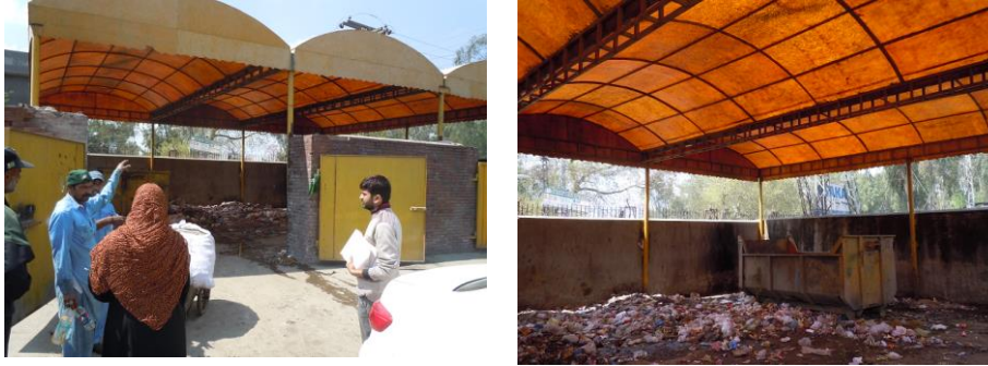
Photo 2.3.4 Current Situation of Waste Collection in General Bus Station
