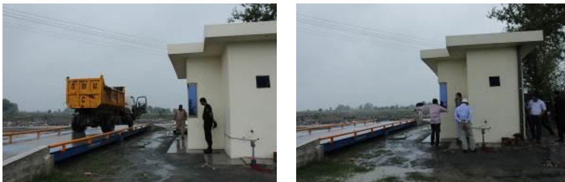
Photo 2.3.7 Installed Weighbridge at Gondlanwala
