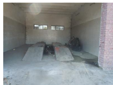
Photo 2.3.1 Current Situation of Vehicle Workshop
