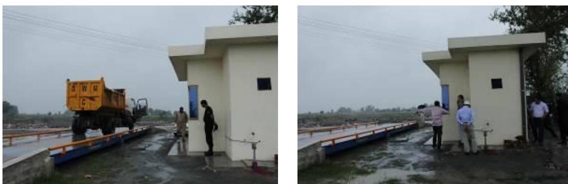
Photo 2.3.3 Installed Weighbridge at Gondlanwala
