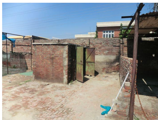
Photo 2.9.2 Storeroom for Waste at a Hospital
