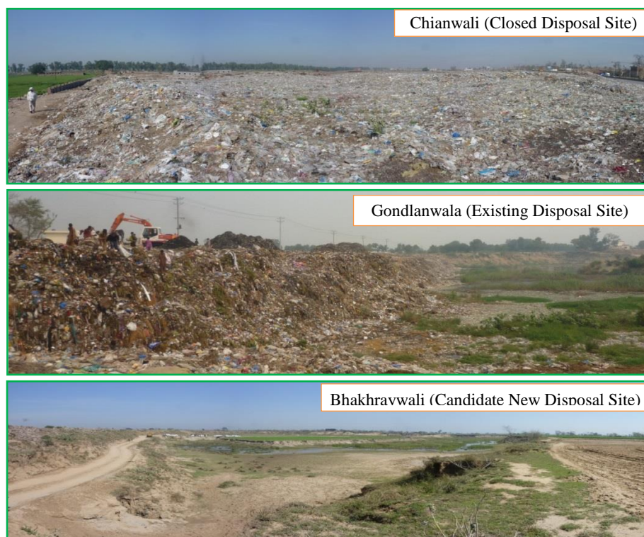
Photo C.2.1 Current Status of Final Disposal Sites
