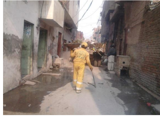
Figure 20: Holland-1, Loading from a Street having drainage Problem
